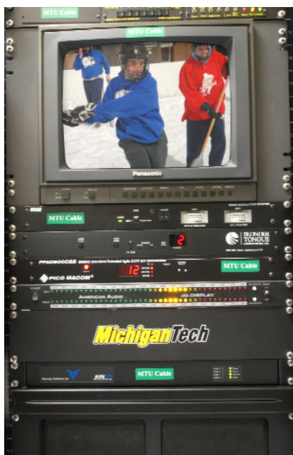
An AVN210 encoder in one of Michigan Tech's data centers, streaming video out to Internet2
